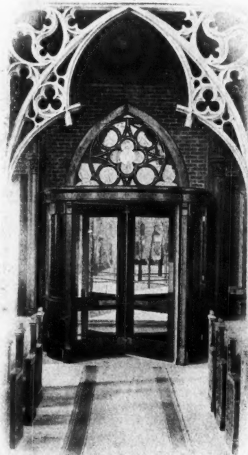
VAN KANNEL REVOLVING DOOR John's German Evangelical Lutheran Church, Passaic, N. J.
