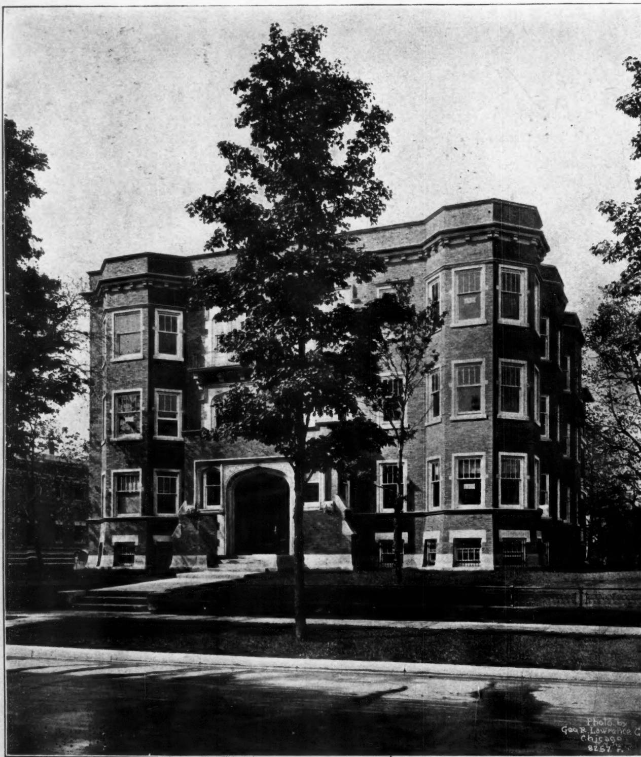
APARTMENT BUILDING, CHICAGO
