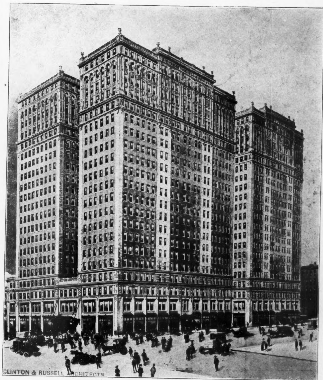
CHURCH STREET TERMINAL BUILDINGS. HUDSON & MANHATTAN RAILROAD CO., NEW YORK Clinton & Russell, Architects
