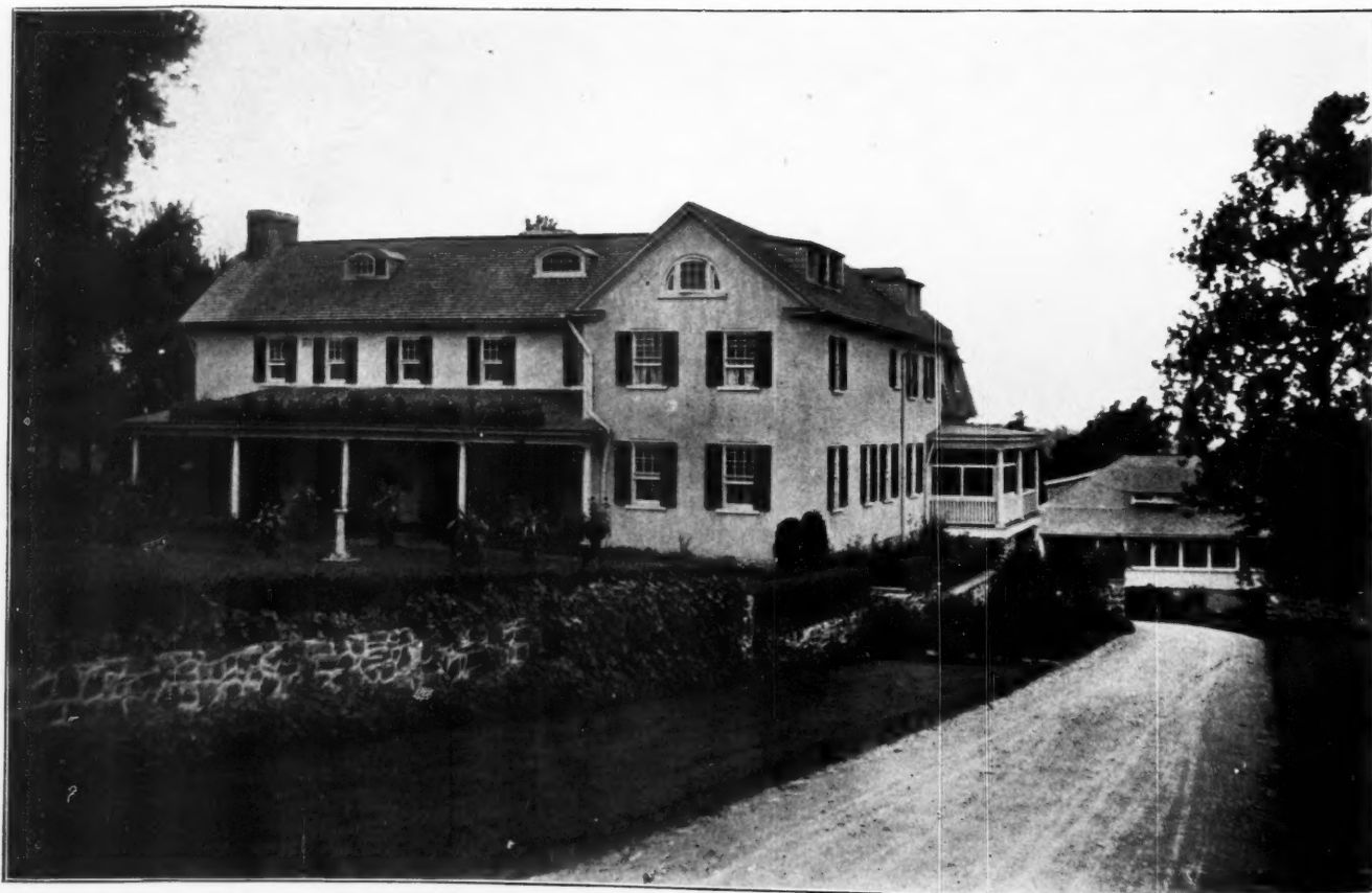
ALTERATIONS AT "WESTFIELD," VILLA MORA
