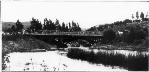
A GRACEFUL LITTLE BRIDGE.
