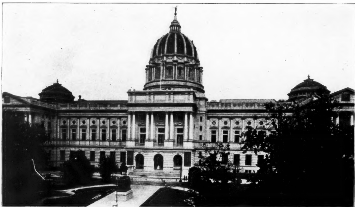
THE STATE CAPITOL, HARRISBURG, PENNSYLVANIA Jos. M. Huston, Architect
