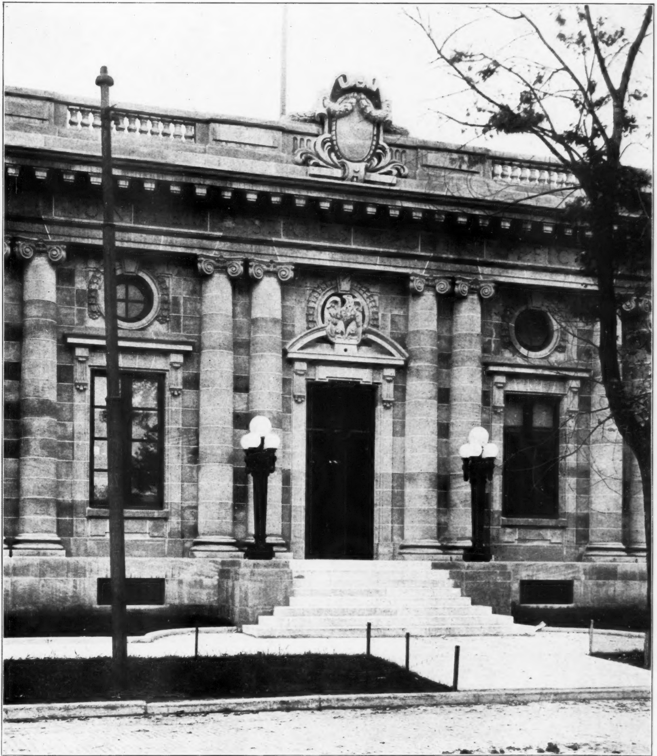
ENTRANCE DETAIL. U. S. POSTOFFICE. EVANSTON, ILL. J. Knox Taylor, Supervising Architect
