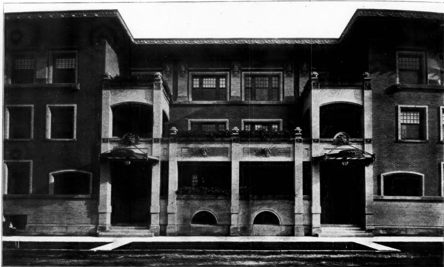
DETAIL VIEW, THE LOGGIA.
