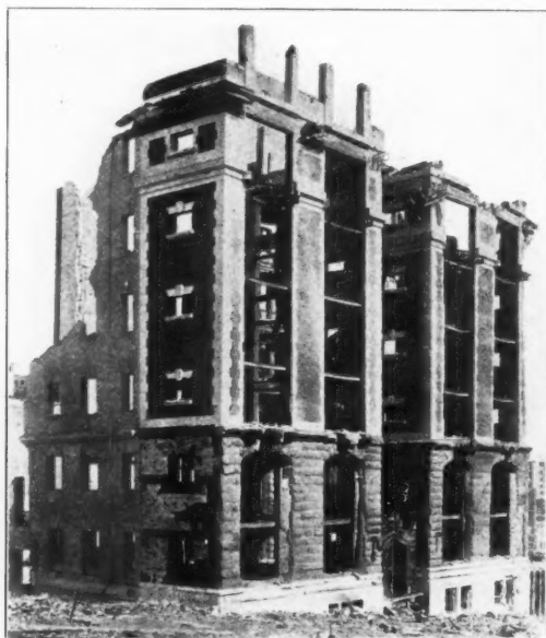
WEST GATE APARTMENTS. STONEWORK DEMOLIALIZED. ENAMELED BRICK UNMARRED.
