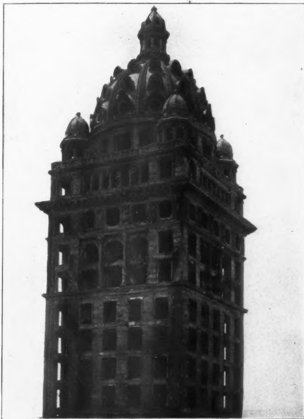
CALL BUILDING. SHOWING DAMAGE TO STONework. TERRA COTTA DOME UNINJURED.
