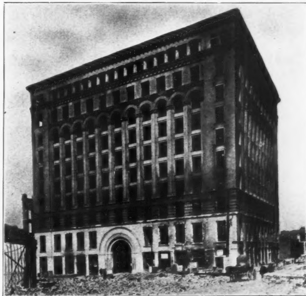
MILLS BUILDING. STONework BADLY SPALLED. EIGHT UPPER STORIES OF BRICK AND TERRA COTTA INTACT.
