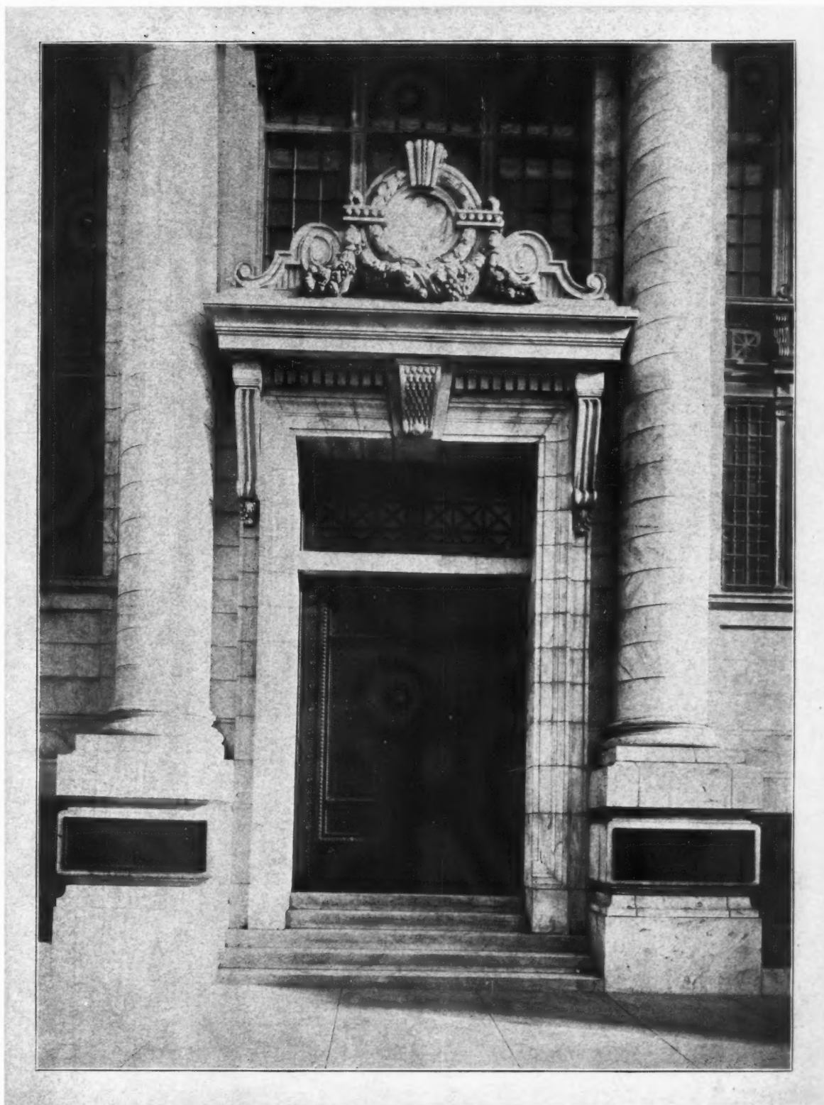
ENTRANCE DETAIL, NATIONAL MECHANICS' BANK, BALTIMORE, MD.
