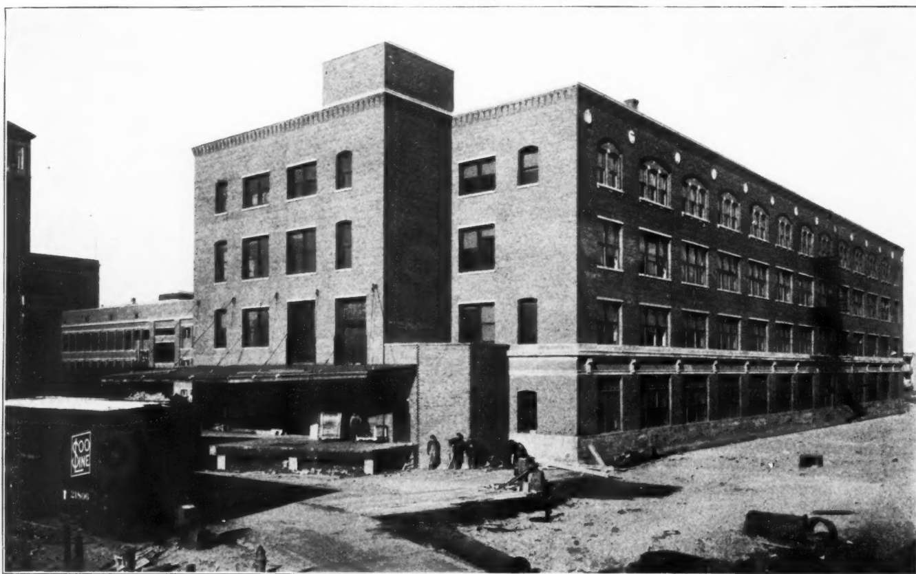
THE PRINTING BUILDING, TRACK VIEW.
