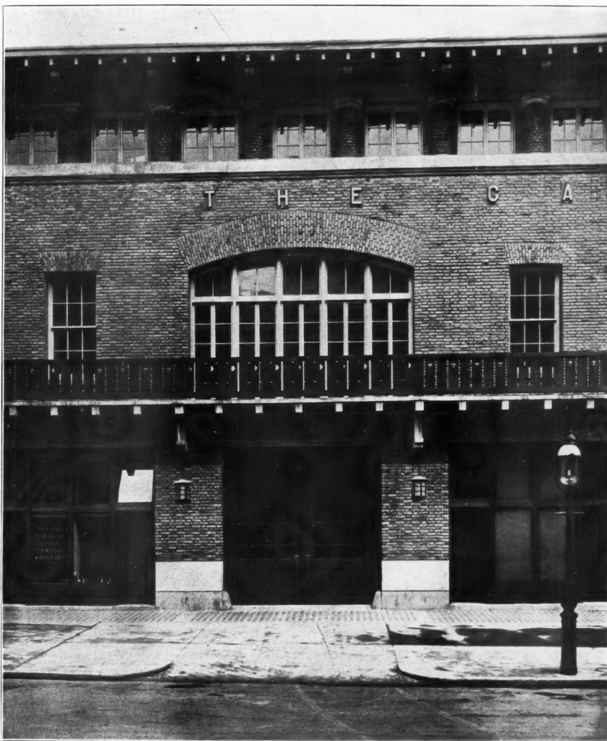
DETAIL VIEW, GARAGE, BALTIMORE, MD.
