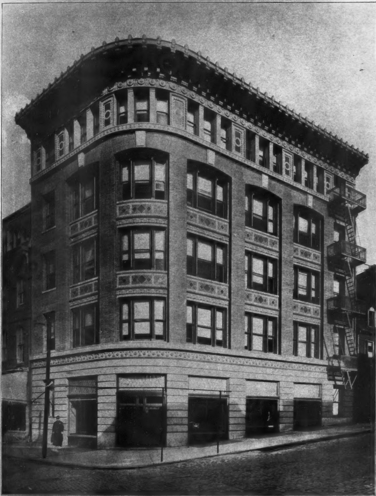
BUILDING FOR CONSOLIDATED GAS CO., BALTIMORE, MD.
