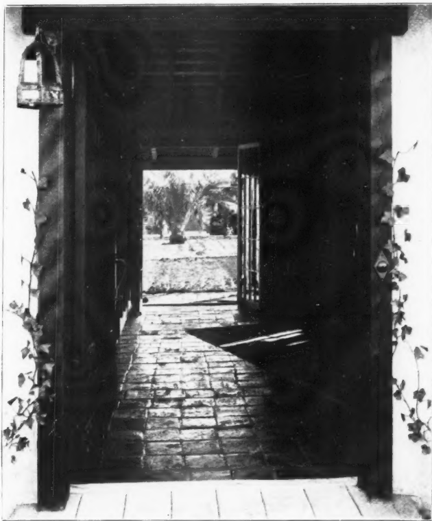
THROUGH FRONT DOOR AND HALL INTO PATIO.
