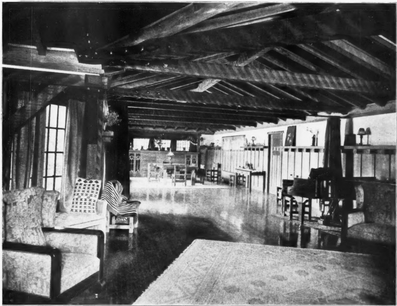
VIEW TOWARDS SOUTH, LIVING ROOM.
