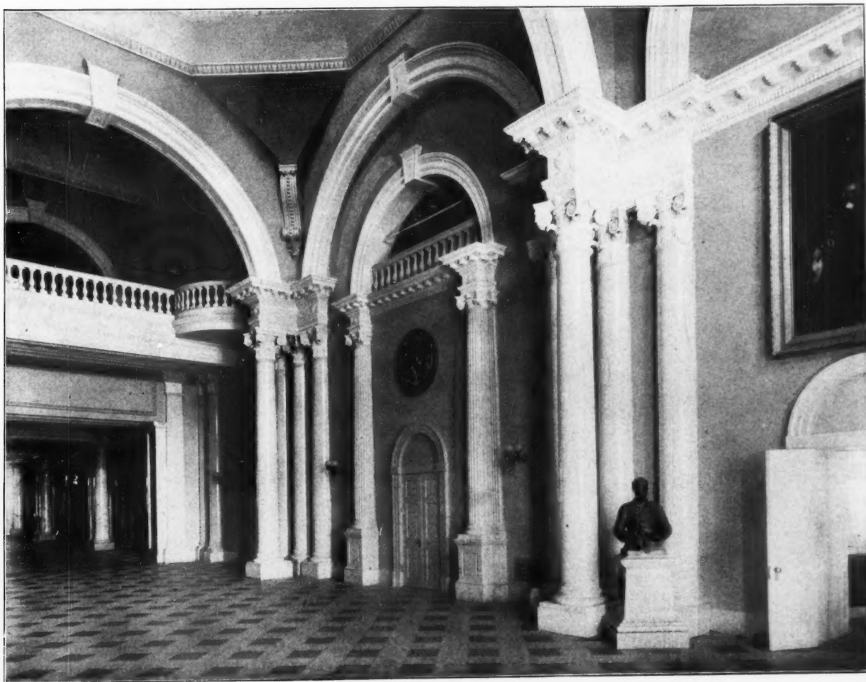
CORRIDOR, OLD BUILDING, VIEW TOWARDS NEW ANNEX.
