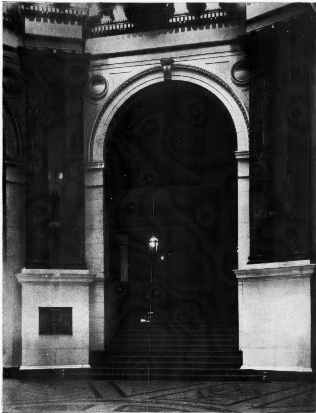
VIEW IN ROTUNDA, CHICAGO POST OFFICE.
