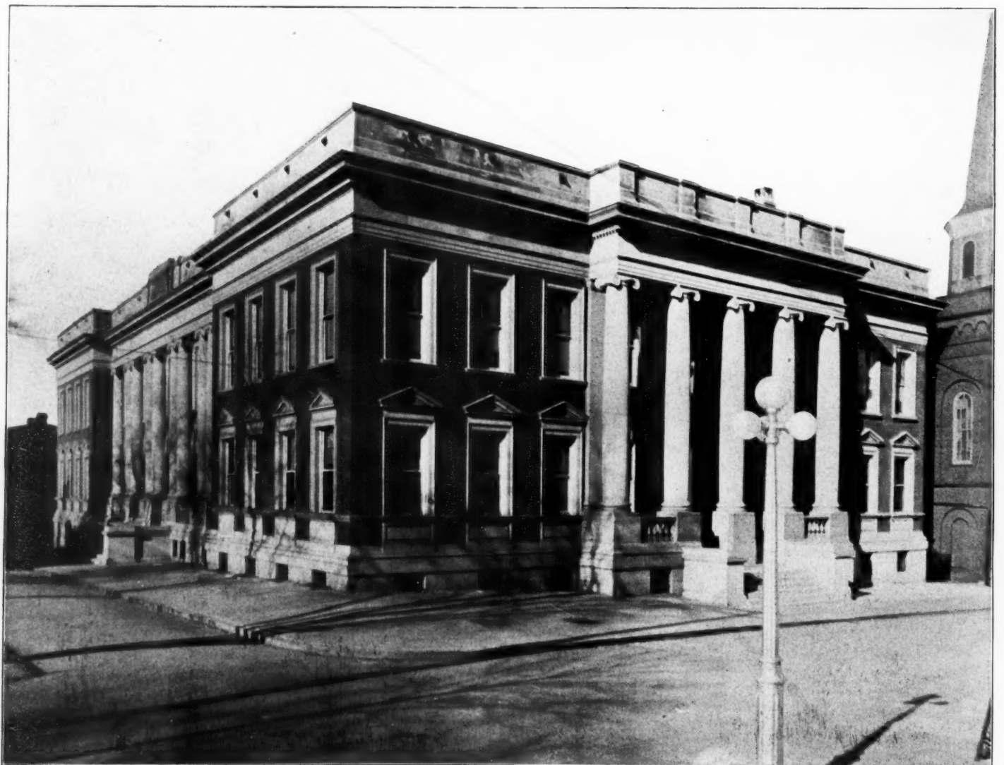
COURT OF APPEALS BUILDING, ANNAPOLIS, MD. BALDWIN & PENNINGTON, ARCHITECTS, BALTIMORE.
