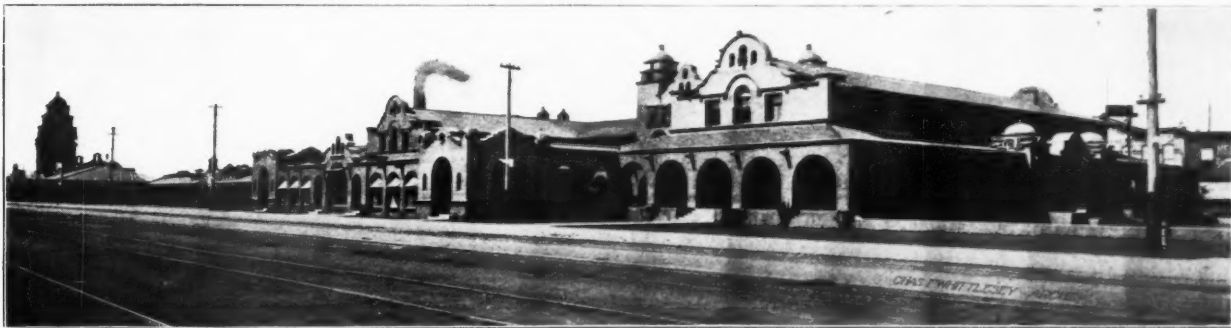
STATION AND HOTEL FOR SANTA FE RAILWAY, AT ALBUQUERQUE, N. M.
