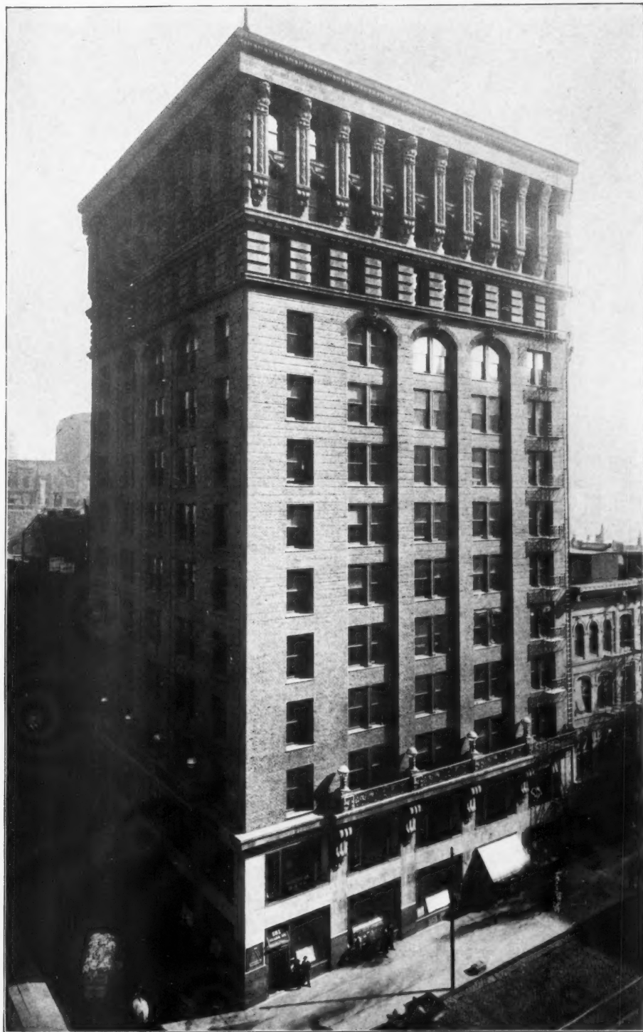
THE RECTOR BUILDING, CHICAGO JARVIS HUNT, ARCHITECT
