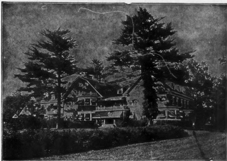
RESIDENCE ON THE ESTATE OF THE LATE WM. C. WHITNEY, LONG ISLAND, N. Y.
