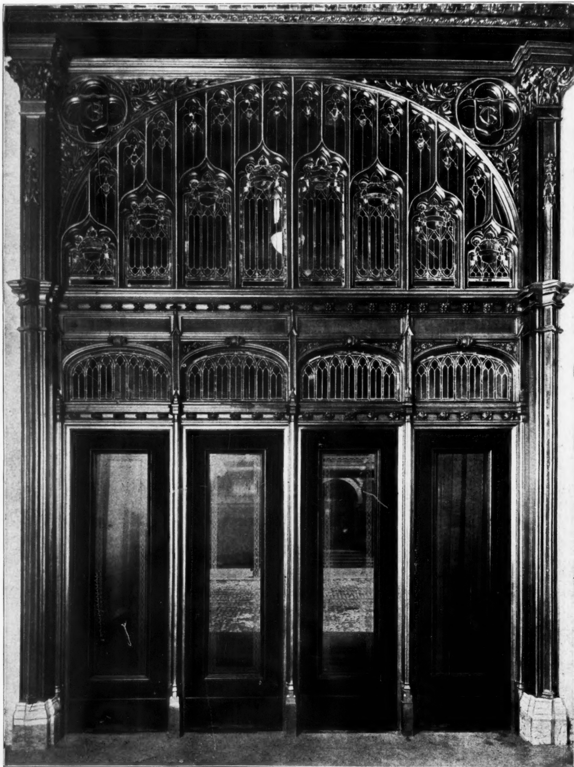
BRONZE VESTIBULE SCREEN, TRINITY BUILDING, NEW YORK.
