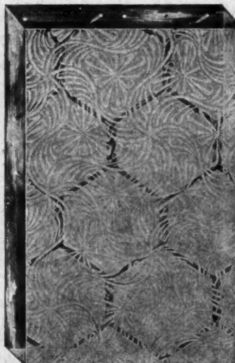
Maze Wire Glass in elevator enclosures.
