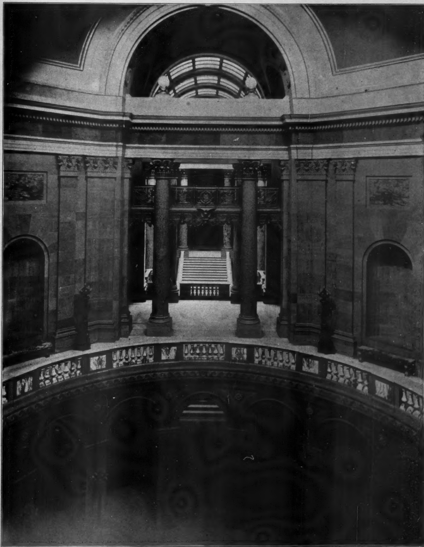
VIEW ACROSS ROTUNDA. SECOND FLOOR TOWARDS SENATE CHAMBER NEW MINNESOTA CAPITOL BUILDING, ST. PAUL CASS GILBERT, ARCHITECT
