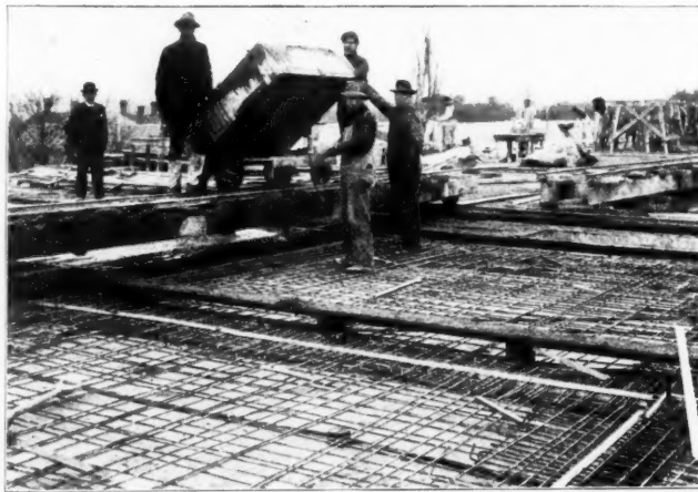
VIEW SHOWING JOINING OF CONCRETE
