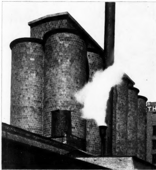
HOLLOW TILE GRAIN ELEVATOR, AT CHICAGO
