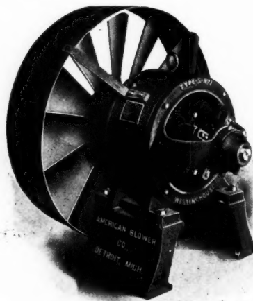
Westinghouse Type S Motor Driving Fan
