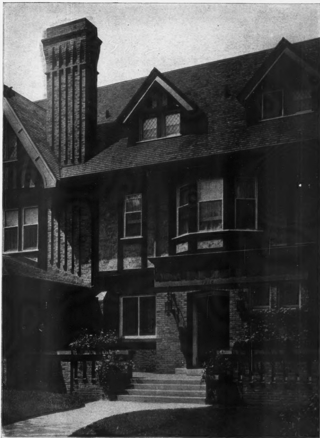
ENTRANCE DETAIL, HOUSE OF F. E. FRENCH, EVANSTON, ILLS.
