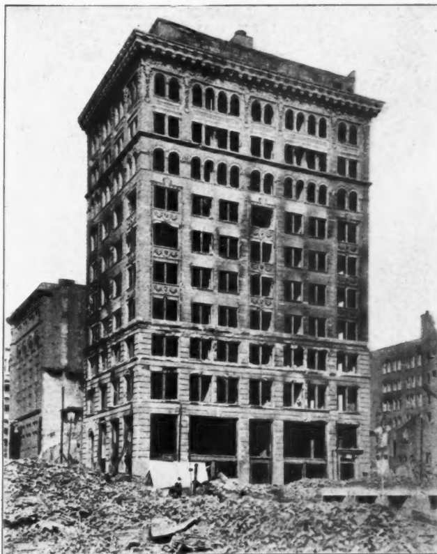
UNION TRUST BUILDING. (Note condition of stonework.)
