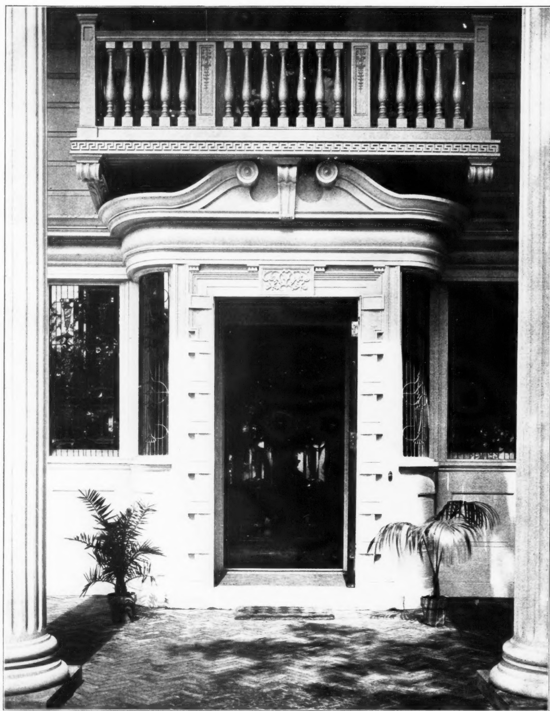
ENTRANCE DETAIL, RESIDENCE OF C. A. WARD, EVANSTON, ILL.
