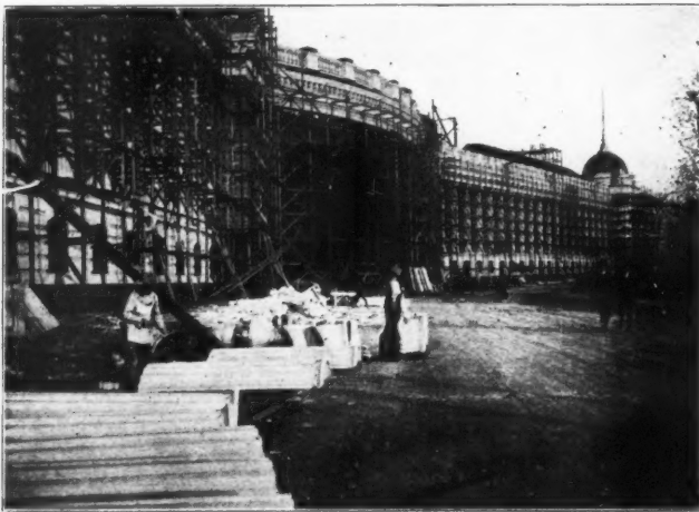
SOUTH SIDE OF THE VARIED INDUSTRIES BUILDING, UNDER CONSTRUCTION.
