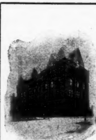
MAIN BUILDING ARMOUR INSTITUTE.
