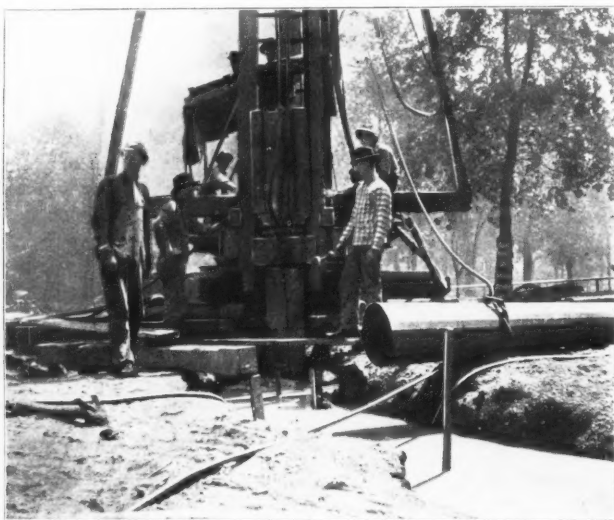
CORE COLLAPSED READY TO BE WITHDRAWN.
