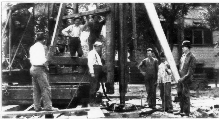
PILE-CORE WITHDRAWN AND READY TO RECEIVE ANOTHER SHELL.
