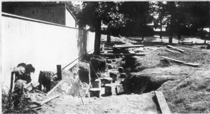
CONCRETE PILES READY FOR RECEPTION OF CONCRETE CAP.
