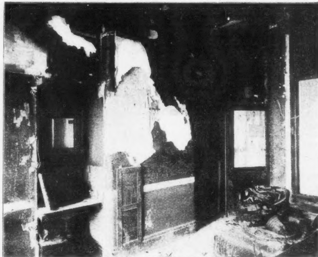
"THOUGH IN SEVERAL PLACES THE PLASTERING HAD FALLEN FROM THE TILE, THE WALLS WERE OTHERWISE INTACT."
