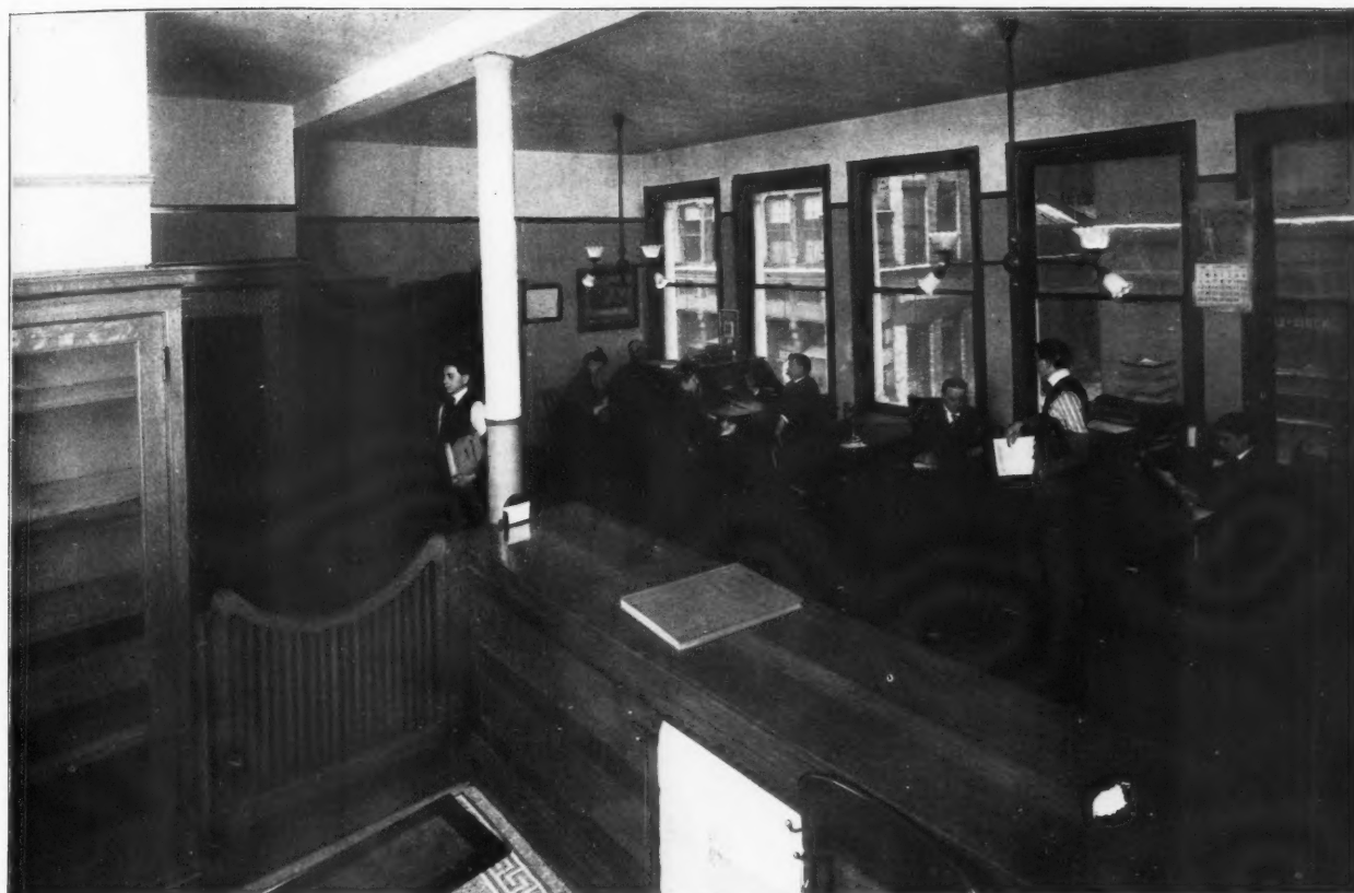
GENERAL OFFICES, SECOND FLOOR.
