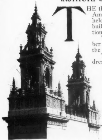
TOWERS OF MACHINERY BUILDING.
