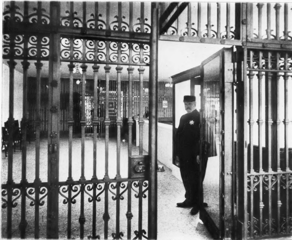
GENERAL VIEW OF ENTRANCE TO GREAT VAULTS, GUARDED BY DOUBLE SET OF BRONZE GRILLES.
