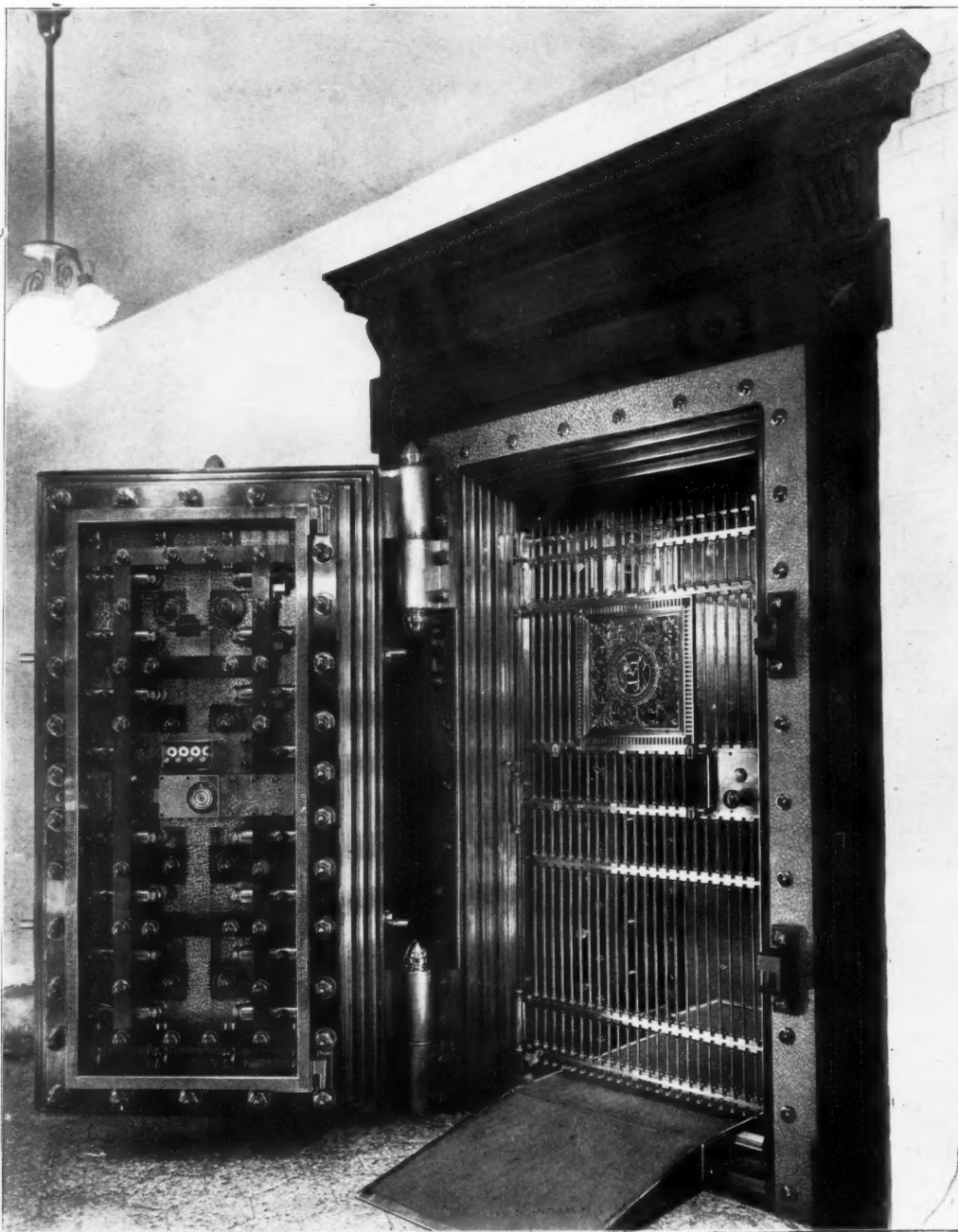
VIEW OF MECHANISM OF OPENED DOOR OF THE GREAT SAFE DEPOSIT VAULTS.
