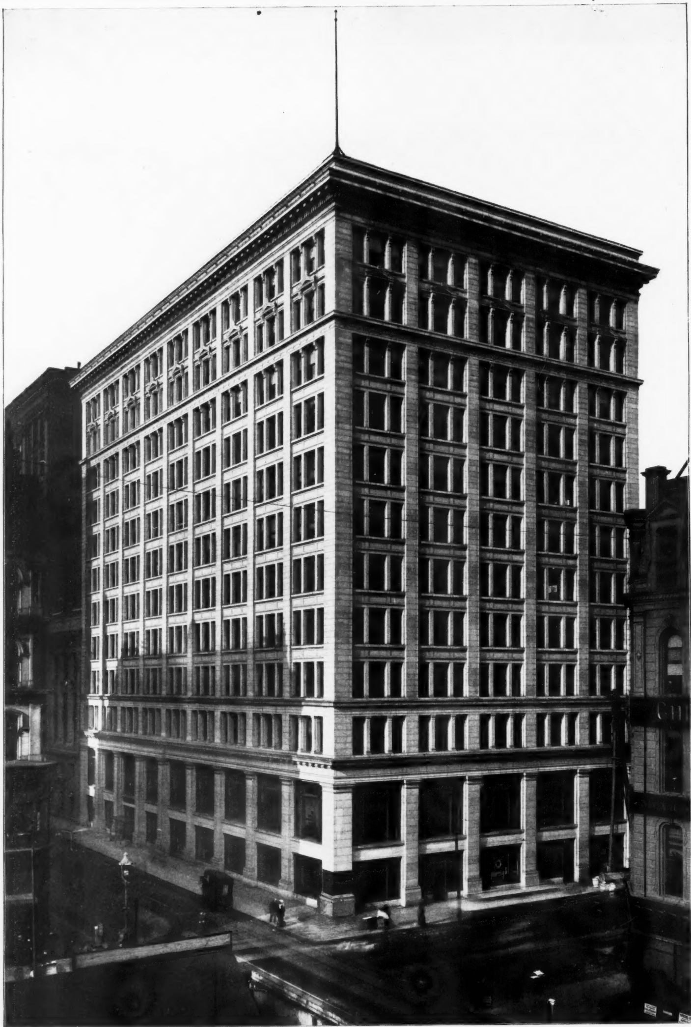
GENERAL EXTERIOR VIEW OF MERCHANTS' LOAN AND TRUST COMPANY BANK BUILDING.
