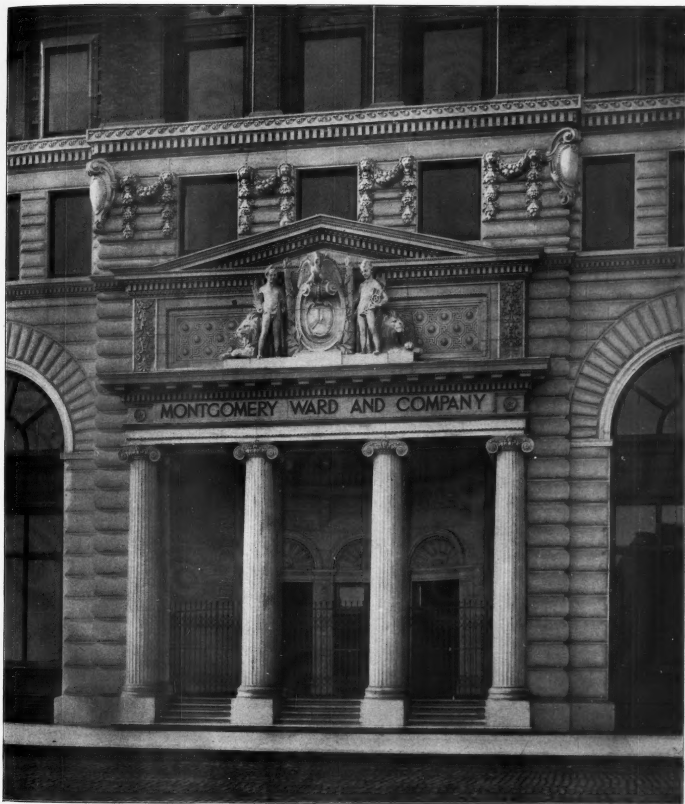
ENTRANCE DETAIL, MONTGOMERY WARD & CO. BUILDING, CHICAGO.
