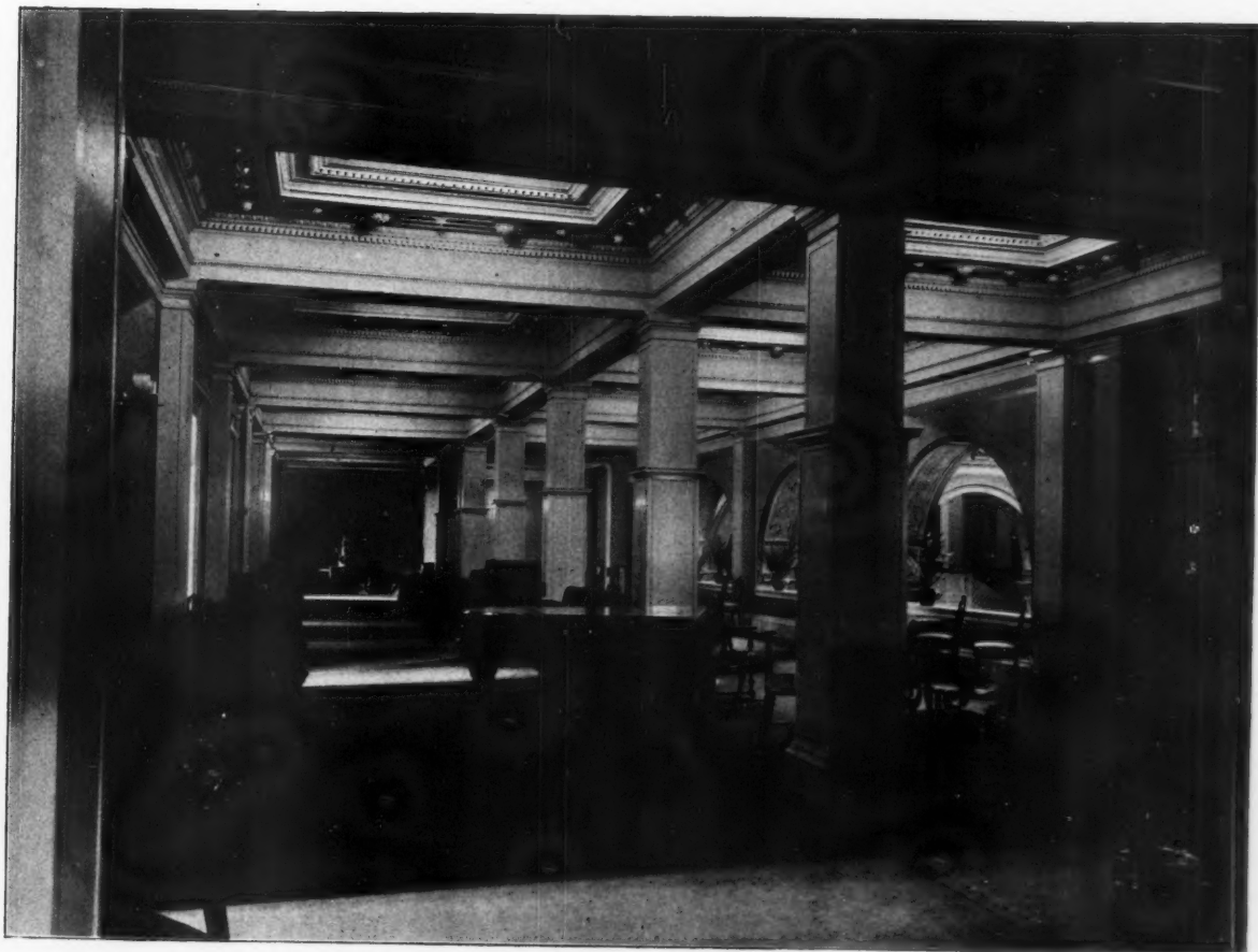
VIEW IN OFFICE.
