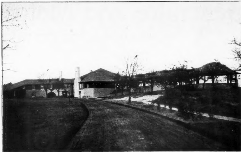
SADDLE AND CYCLE CLUB, EDGEWATER, ILLINOIS. JARVIS HUNT, ARCHITECT, CHICAGO.
