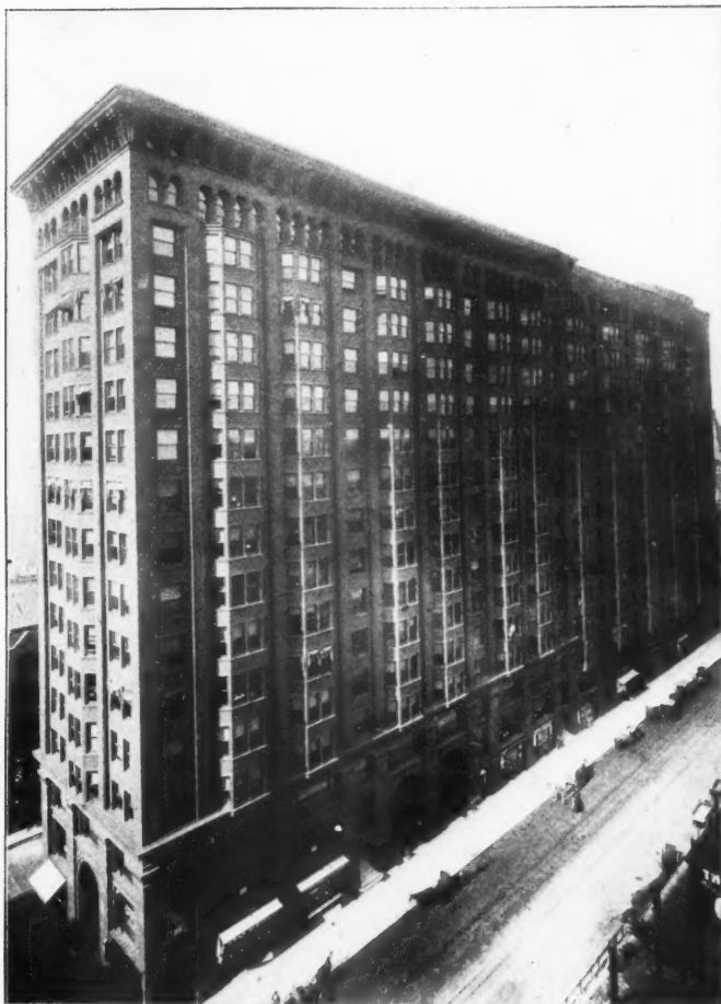
MONADNOCK BUILDING, CHICAGO. Holabird & Roche, Architects. Burnham & Root, Architects.
