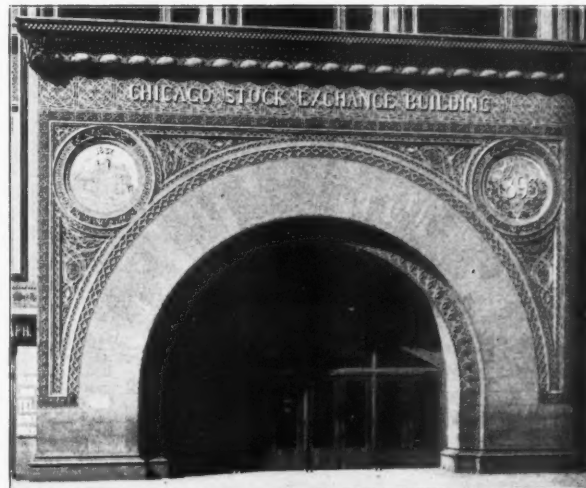
Executed in Terra-cotta by Northwestern T. C. Co. Adler & Sullivan, Architects.
