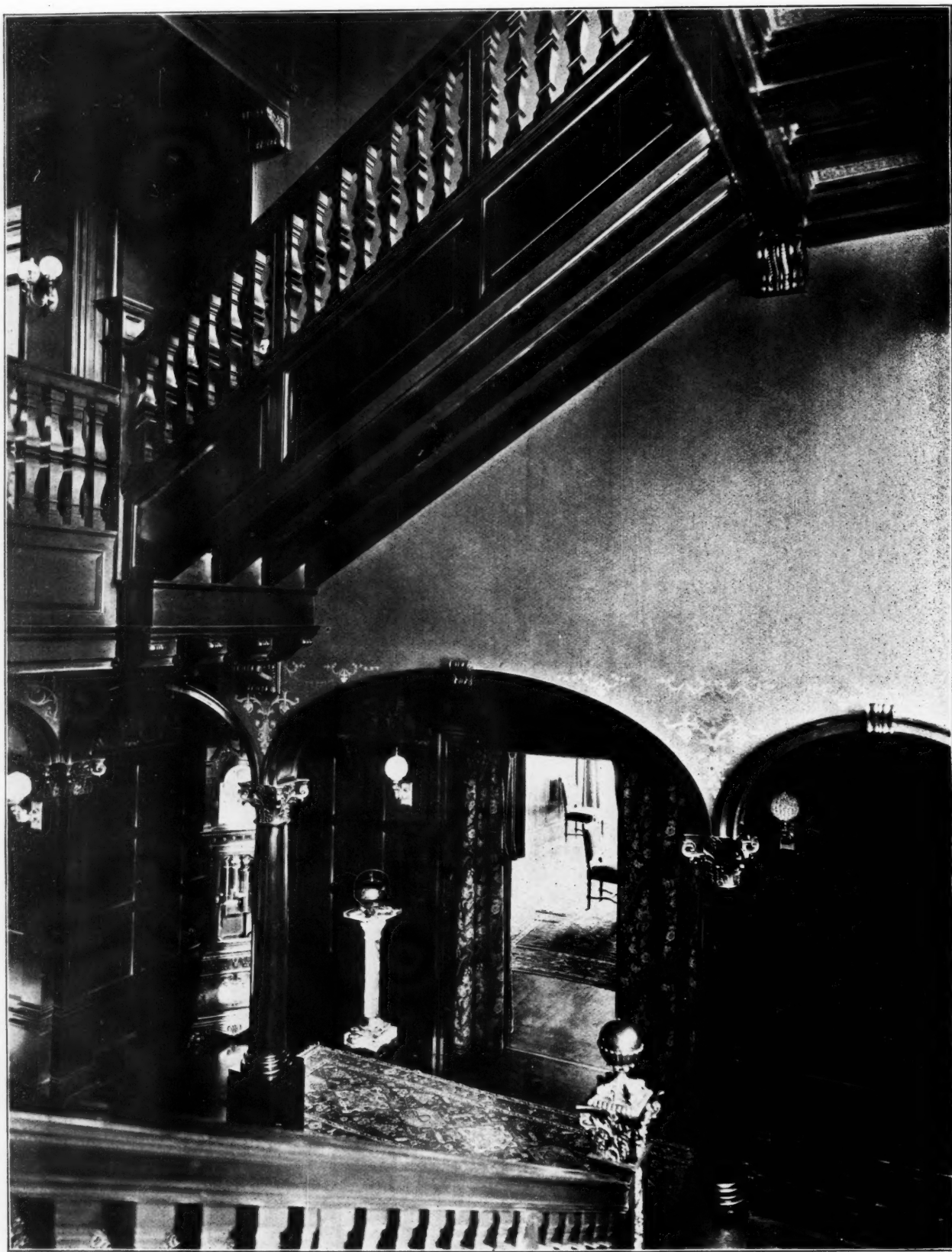
VIEW OF STAIRWAY, VANDERGRIFT RESIDENCE, PITTSBURG, PENNSYLVANIA.
