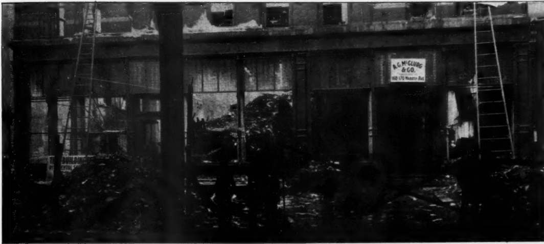
WABASH AVENUE SIDE, SHOWING EFFECT OF FIRE AND LUXFER PRISMS.
