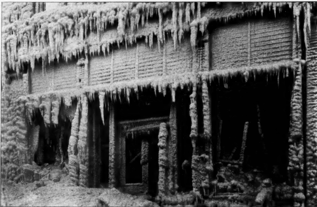
MADISON STREET ENTRANCE, SHOWING LUXFER PRISMS COVERED WITH ICE DURING FIRE.
