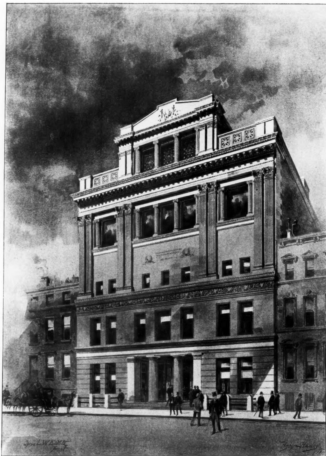
BAR ASSOCIATION BUILDING, NEW YORK. CYRUS L. W. EIDLITZ, ARCHITECT.
