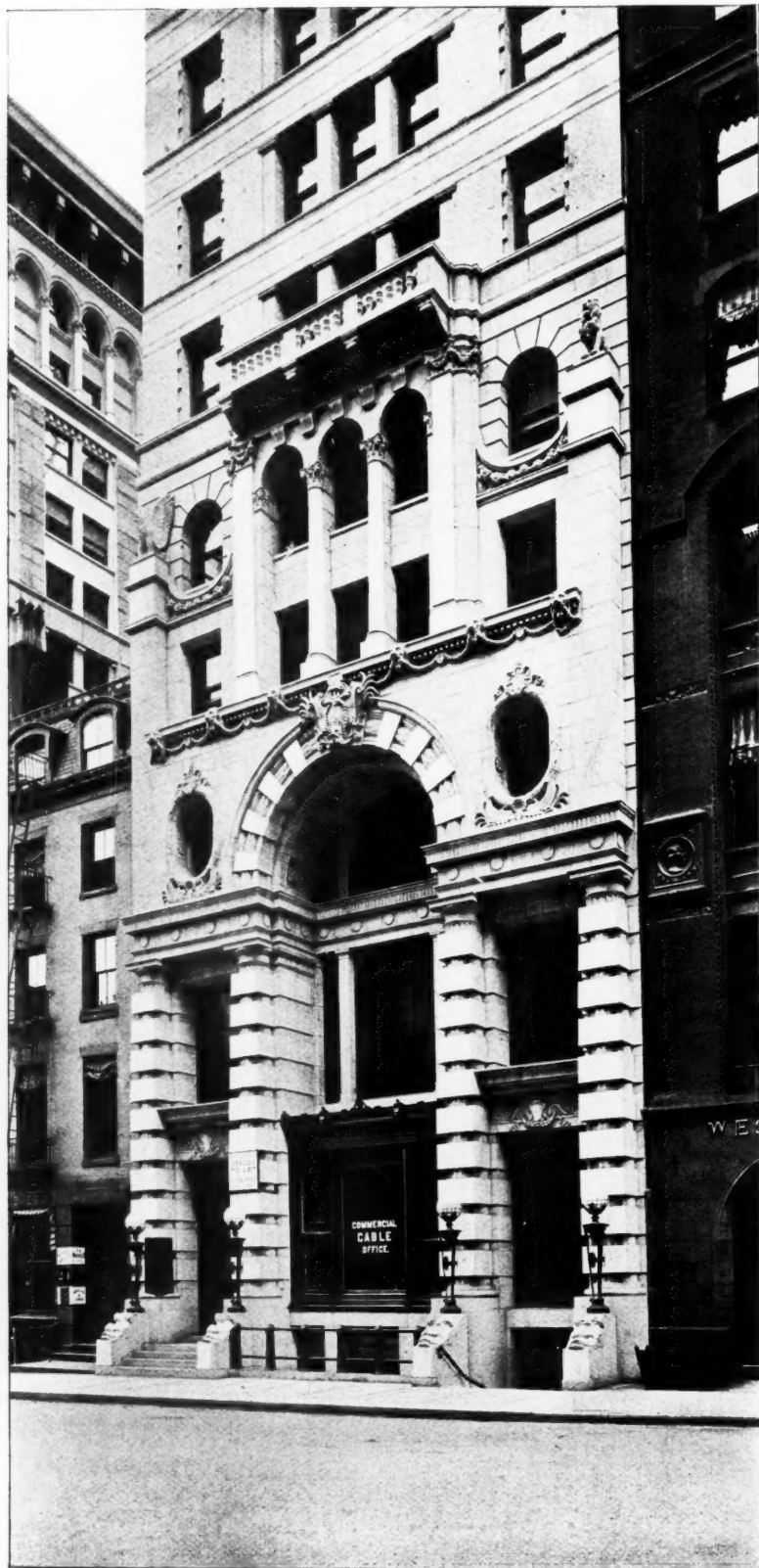
LOWER STORIES, COMMERCIAL CABLE BUILDING, NEW YORK CITY.
