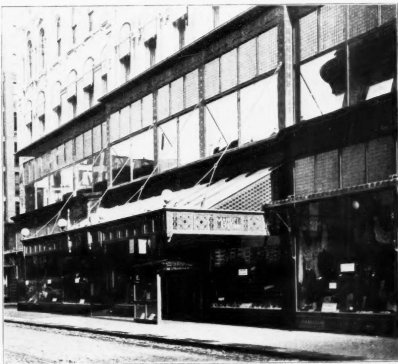
MADISON STREET ENTRANCE.—DETAIL VIEW OF LUXFER PRISMS, CANOPY AND ORNAMENTAL IRON.
