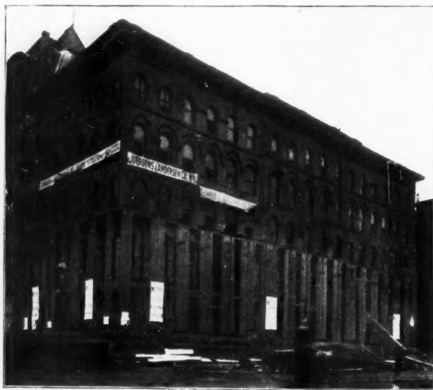
PREPARED FOR REMODELING, SHOWING UPPER STORIES HELD ON JACKSCREWS.
