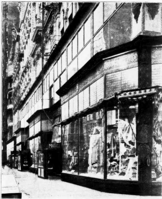
DETAIL VIEW OF STATE STREET FRONT ORNAMENTAL IRON AND LUXFER PRISMS.
