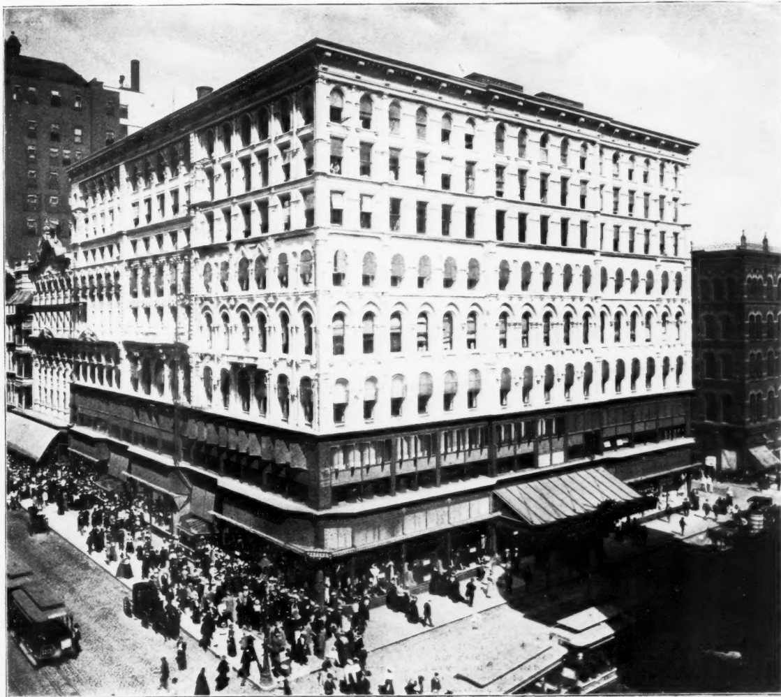
GENERAL VIEW, SHOWING REMODELING WITH ORNAMENTAL IRON AND LUXFER PRISMS.
