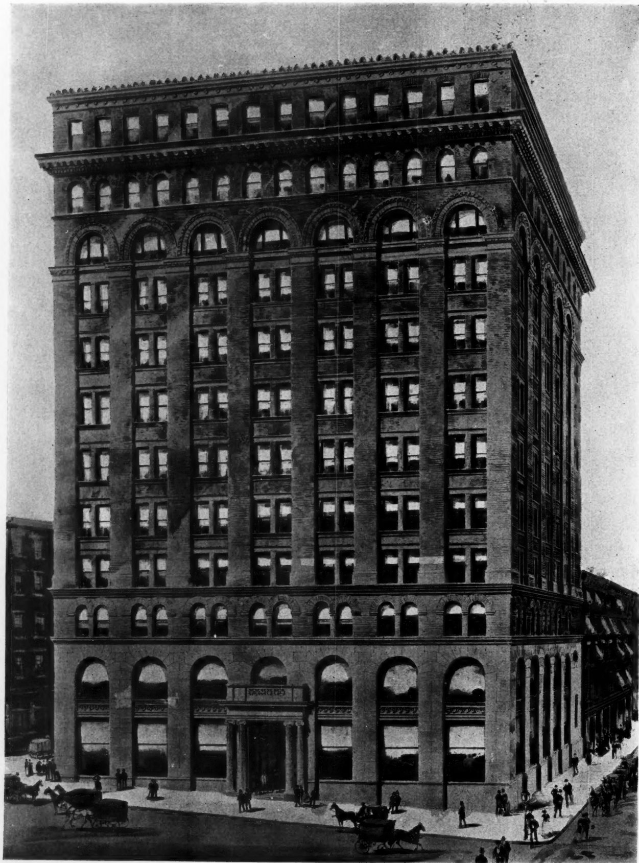
WOODBIDGE BUILDING, NEW YORK.
