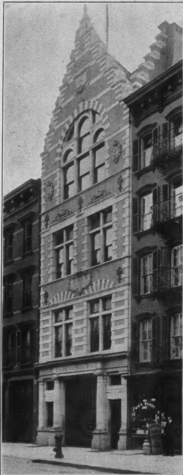
FIRE PATROL BUILDING, NEW YORK CITY.
