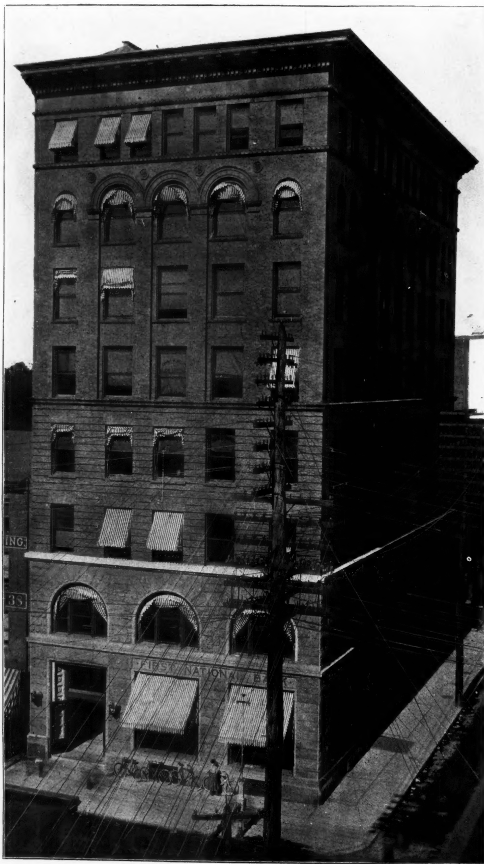
FIRST NATIONAL BANK BUILDING, NEW HAVEN, CONNECTICUT.
