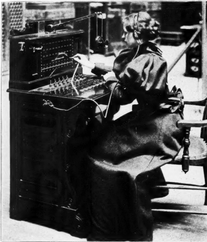
TELEPHONE OPERATING CABINET.
