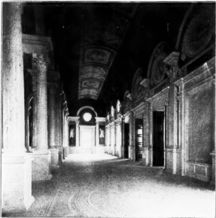
SOUTH VAULT, MAIN HALL, SECOND FLOOR.
