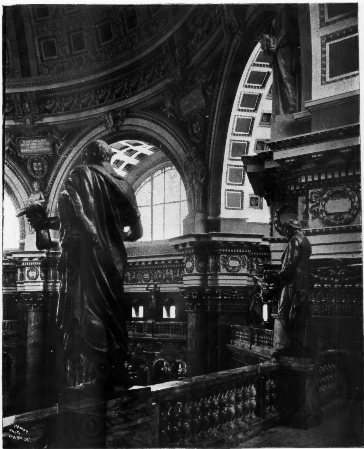
IN THE GALLERY, PUBLIC READING ROOM.
