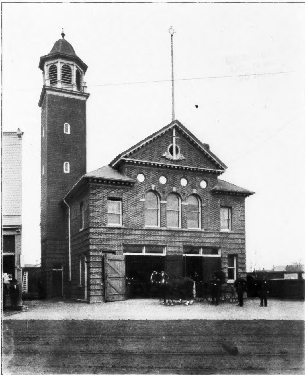
ENGINE HOUSE, DETROIT, MICHIGAN.
