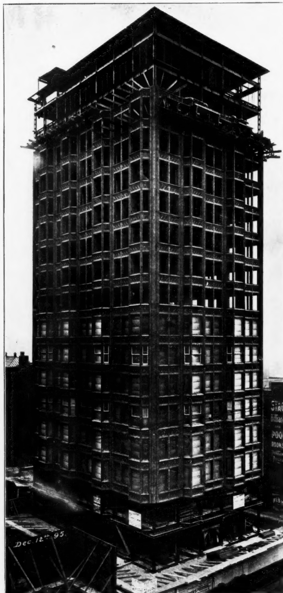
VIEW OF THE BUILDING TAKEN DEC. 12, 1895.
