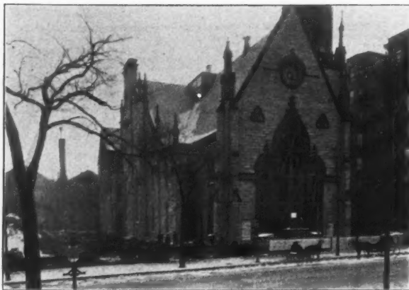
IMMANUEL BAPTIST CHURCH, Showing front bracing, and ready to be moved.
