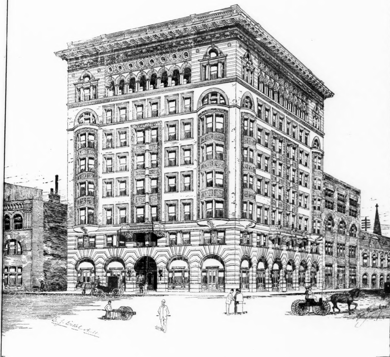
HOTEL BUILDING, ST. JOSEPH, MISSOURI.
