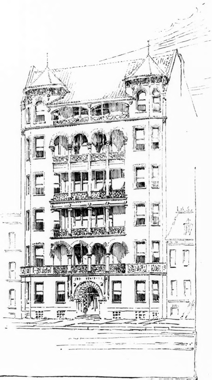
APARTMENT BUILDING, CHICAGO.
