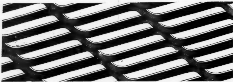
EXPANDED METAL LATH.
