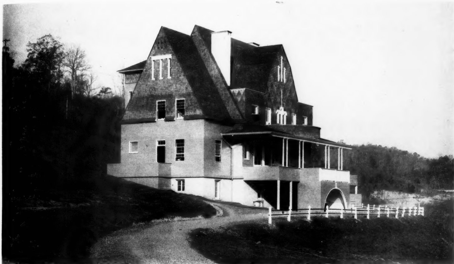
FRONT VIEW, COTTAGE FOR M. E. INGALLS, HOT SPRINGS, VIRGINIA.
