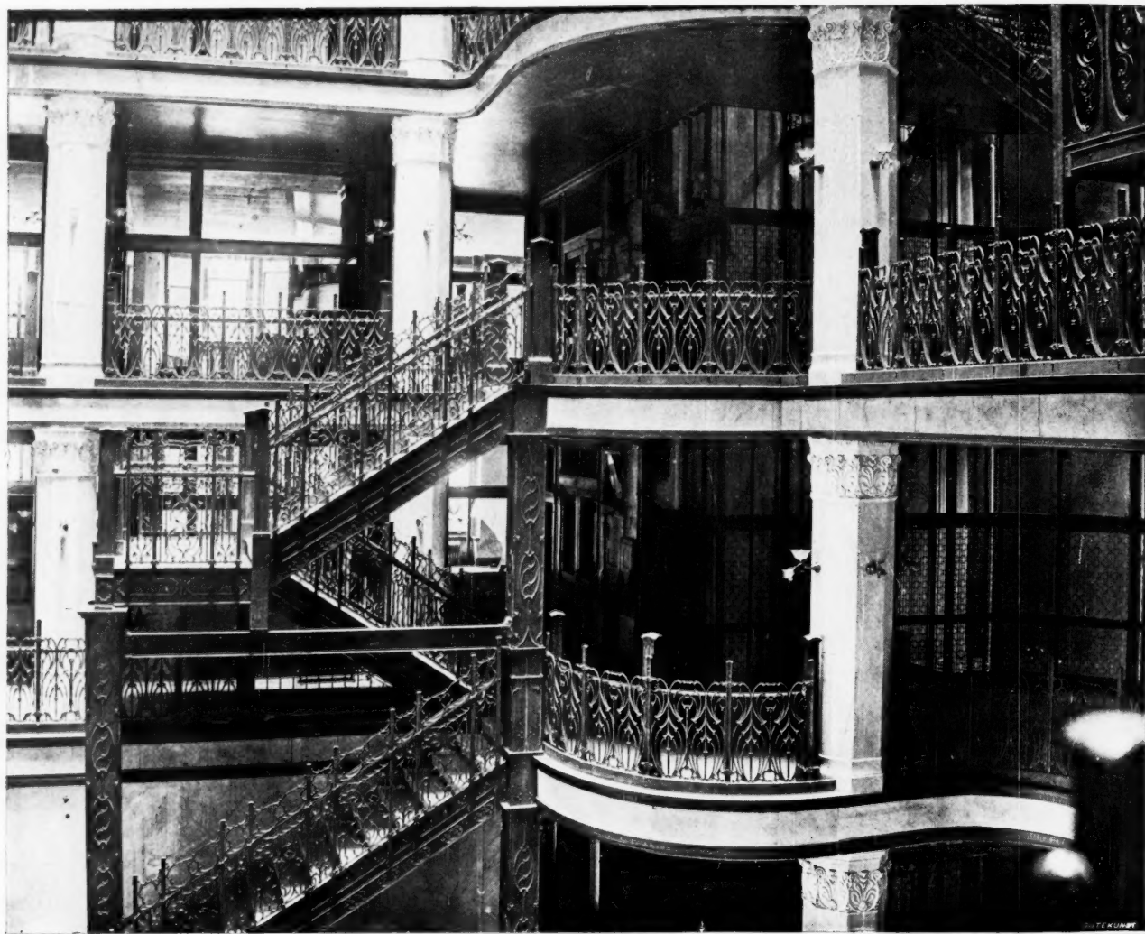
STAIRWAY AND GALLERIES FROM ELEVATORS.
