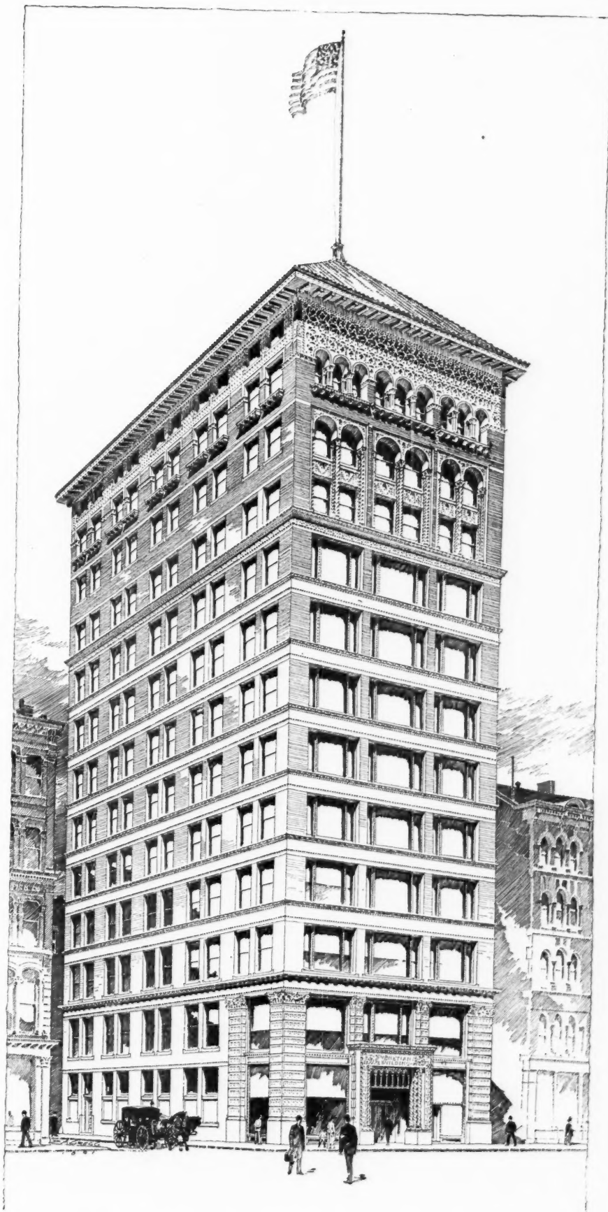
THE VENETIAN OFFICE BUILDING, CHICAGO.
