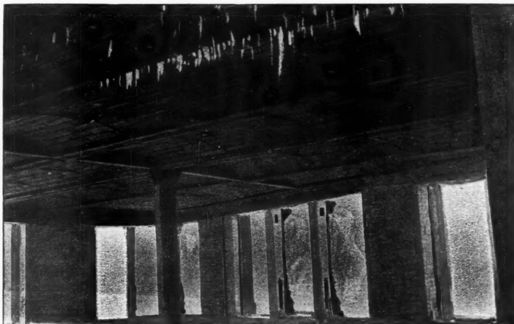
NO. 4.—TENTH FLOOR CEILING IN OLD BUILDING, SHOWING ARCHES UNINJURED AFTER THE FIRE.
