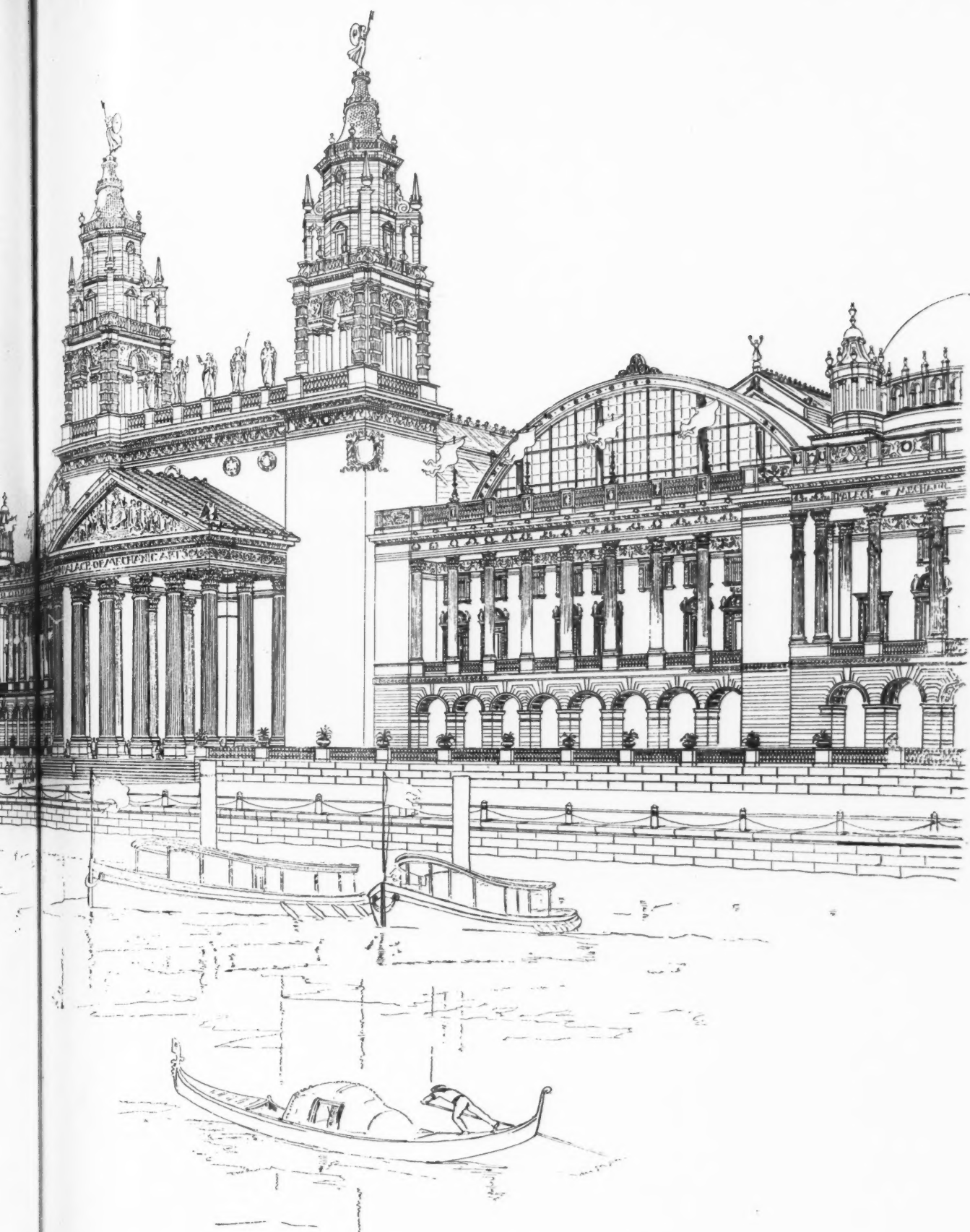
S COLUMBIAN EXPOSITION, CHICAGO. DEPARTMENT OF CONSTRUCTION, MAY, 1891.
